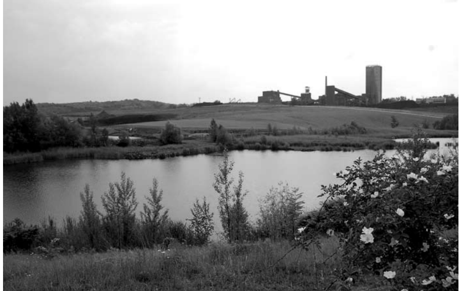
Rehabilitation project – Lazy settling reservoirs in Karviná
